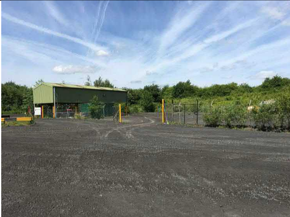
Photograph 15 | Access route to the ash disposal site
