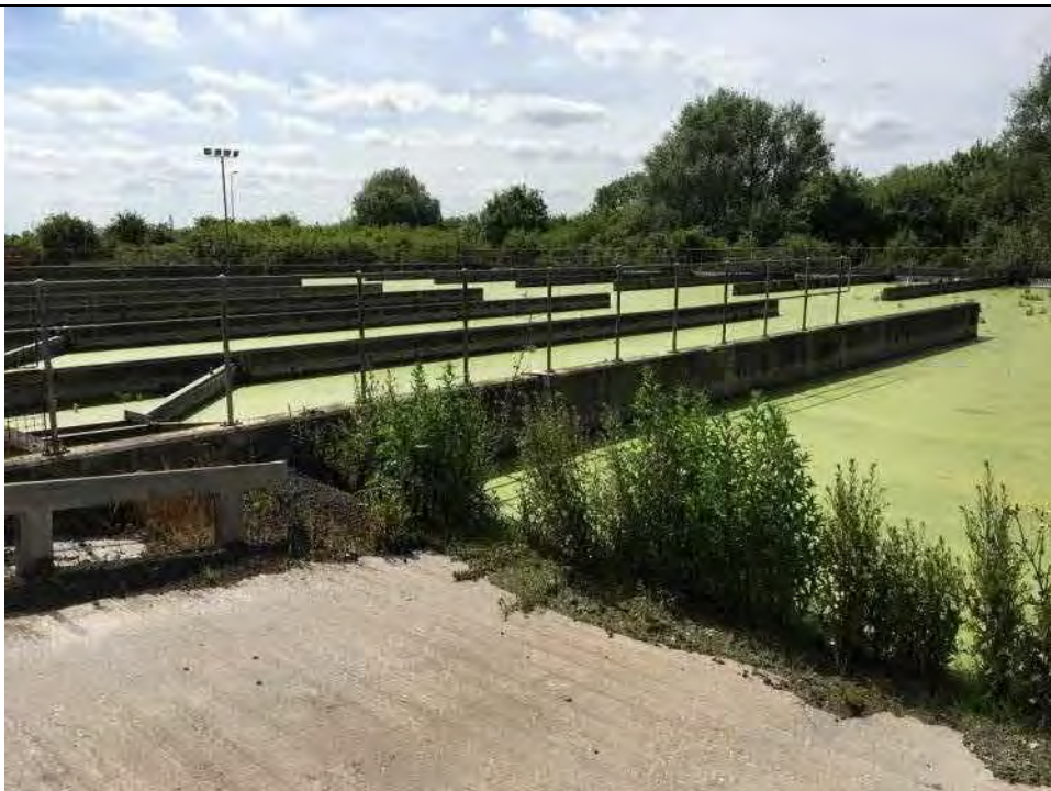
Photograph 24 | Main power station interceptor
