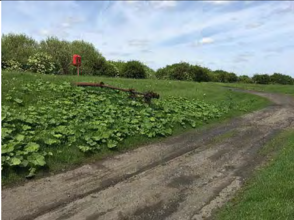
Photograph 23 | Discharge pipe (Source unknown)
