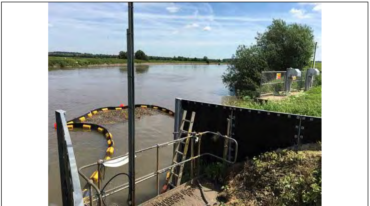
Photograph 26 | River Trent discharge point
