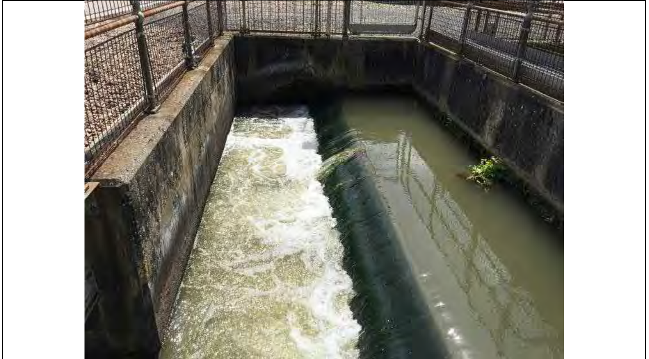
Photograph 25 | Interceptor discharge
