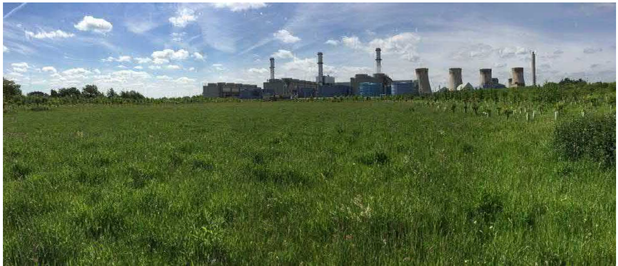
Photograph 20 | Location of Proposed Development (West Burton C) with West Burton B Power Station in background
