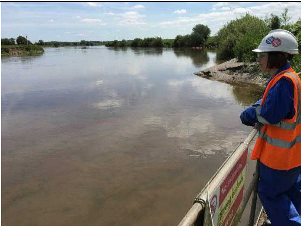
Photograph 28 | Surface water abstraction point
